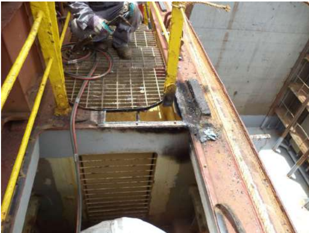
Container ship container section vent repair
