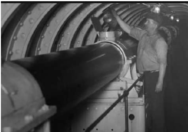
The Shaft Tunnels ( 3 of them) - Greaser Lubricating the bearing(s)
