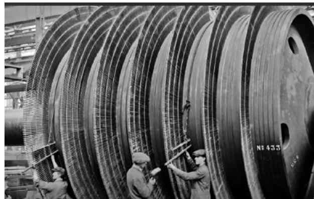
Shows the hundreds of Turbine Blades being installed
