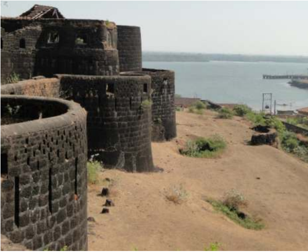
Figure 2 Vijaydurg Fort Bastions
