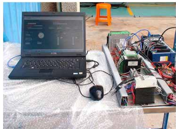
Figure 14. Electrical loading and data acquisition system
