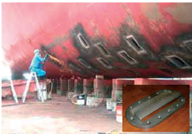
Figure 2. WAIP installation process in dry dock and Cast iron WAIP fitting
