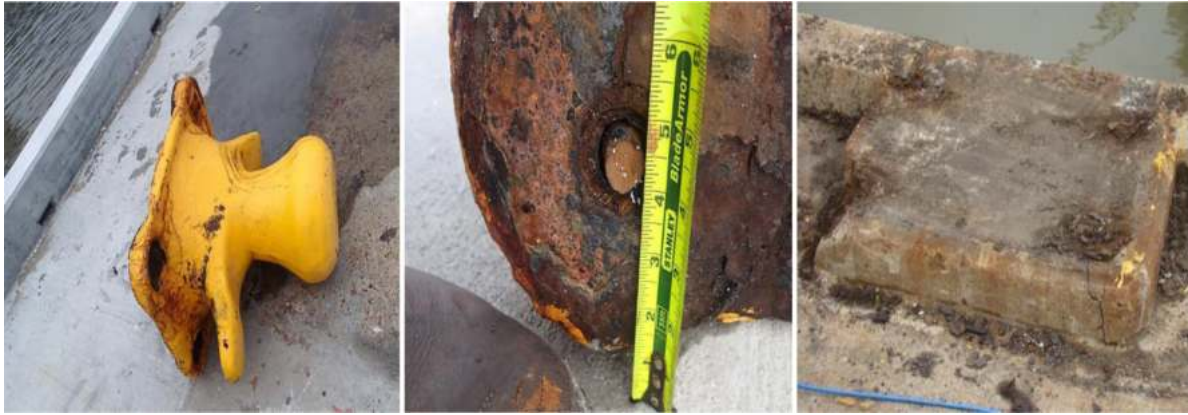
Figure 2. Failed Bollard with failed bolt and damaged concrete base
