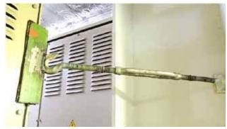
Cargo chain turnbuckle, welded to angle iron, and wedged between the number 1 step-down transformer (left) and a steel beam (right).
