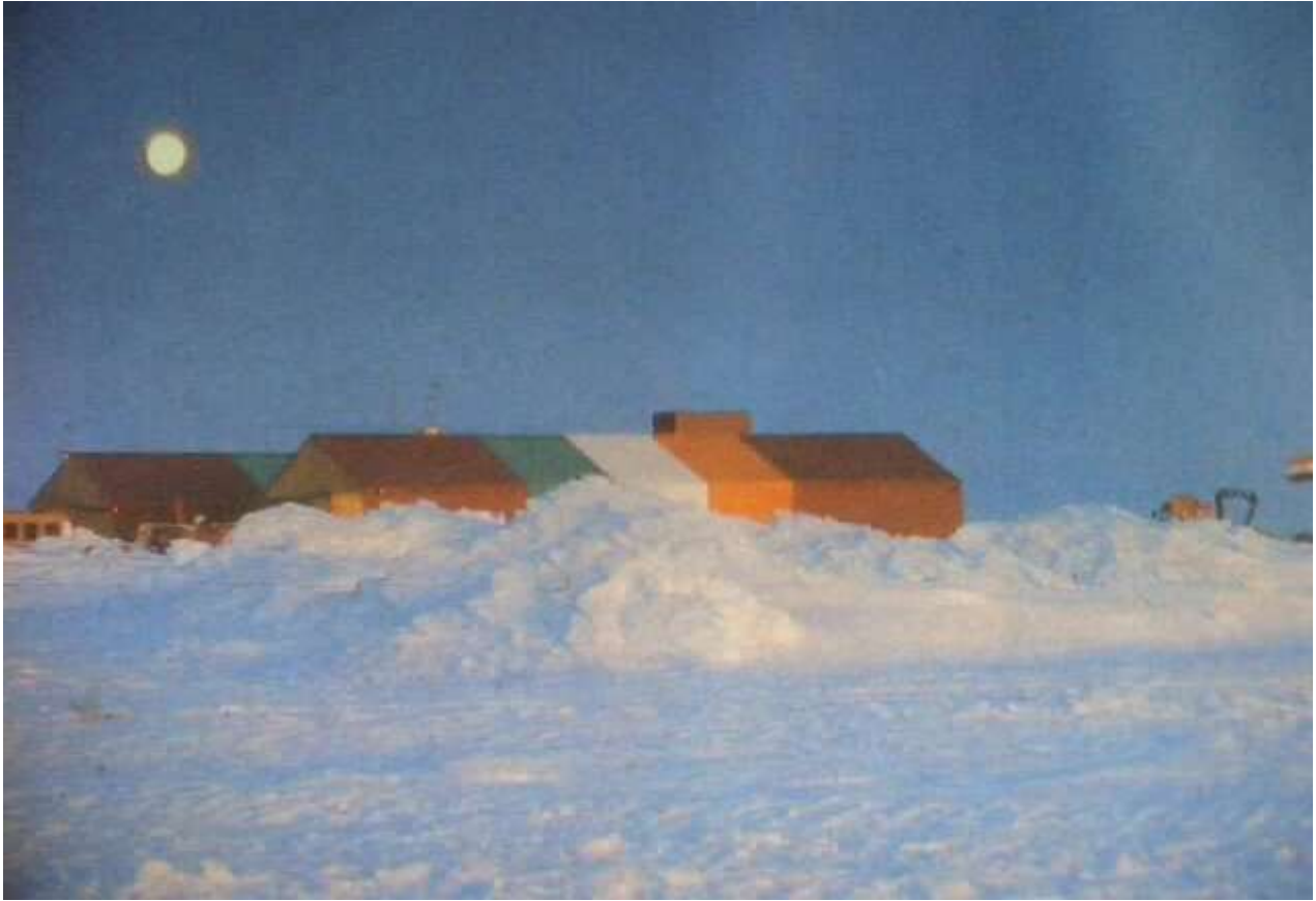
DG station got buried up to roof level in 1987-88
