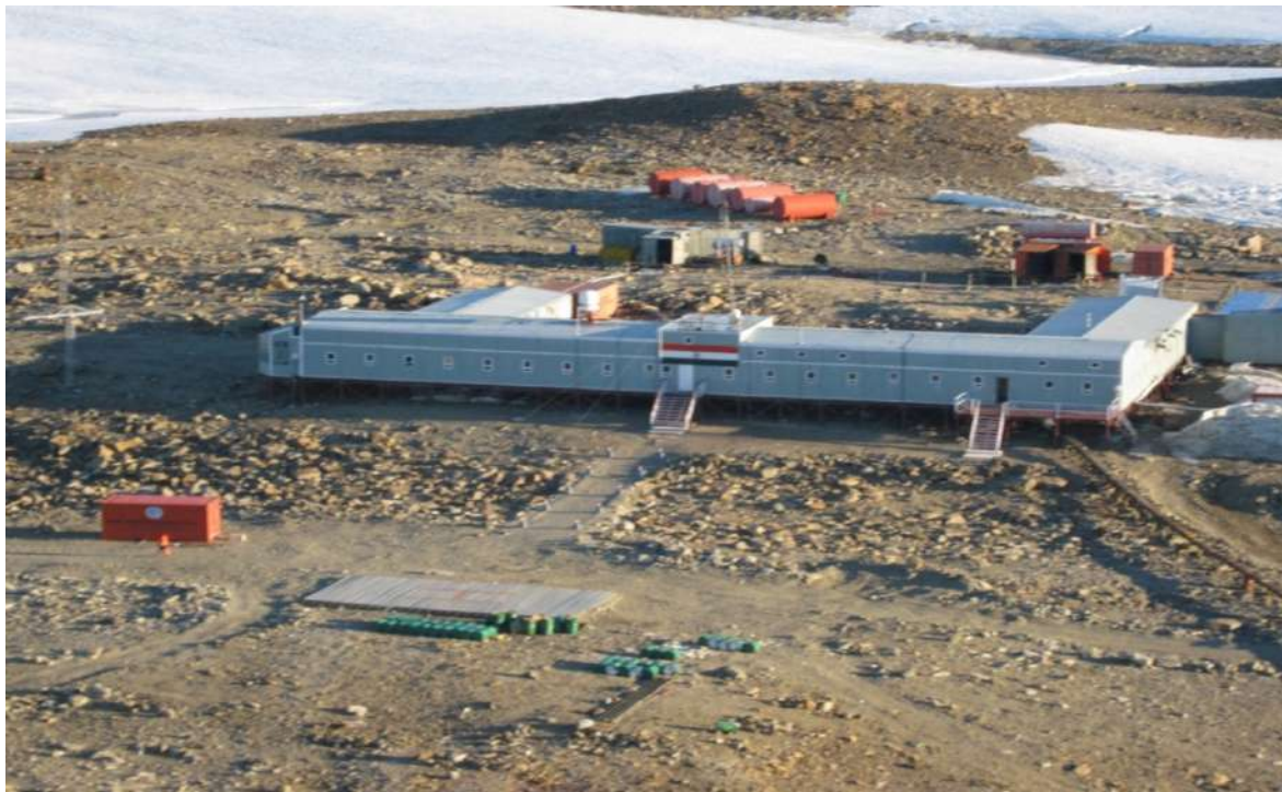
Second station- Maitri-constructed in 1988-89 during summer time
