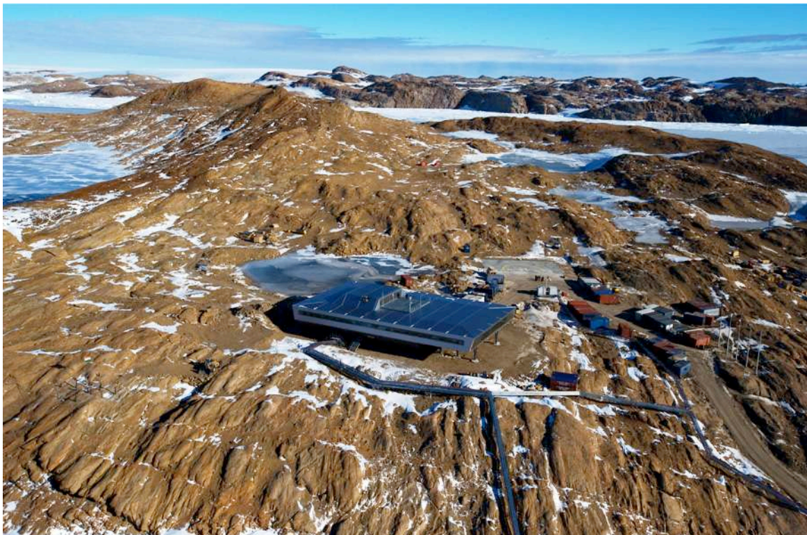
Aerial view of Bharati station at Larsemann hills
