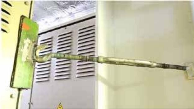
Cargo chain turnbuckle, welded to angle iron, and wedged between the number 1 step-down transformer (left) and a steel beam (right).
