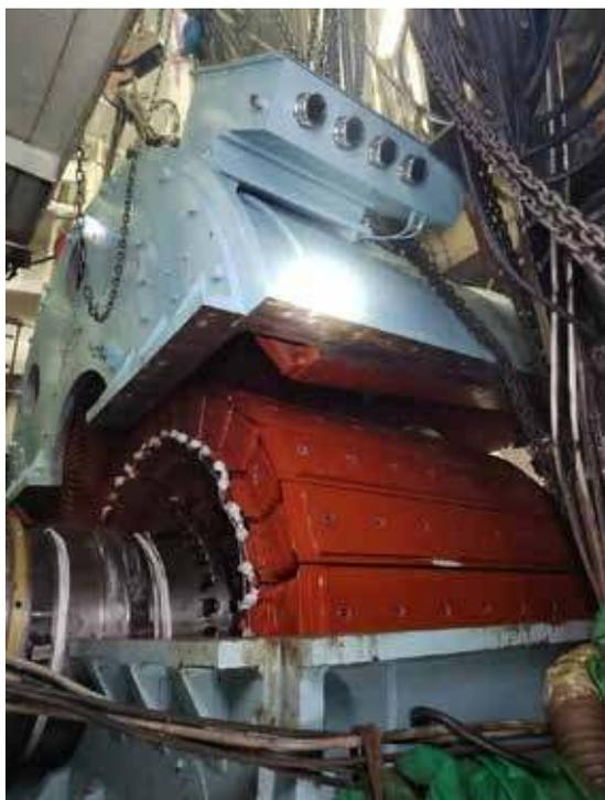
**Figure 2 – Rotor and stator of Shaft generator (courtesy – CSSC/SMDERI)**
