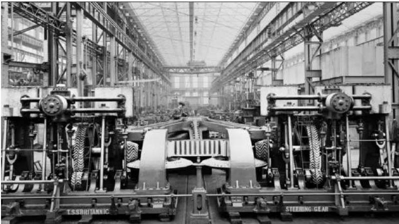
Two Steam Engine on the shop floor, for steering gear
