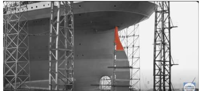
Red shaded portion shows the Rudder Stock
