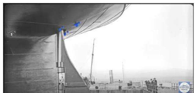
Blue shaded pad eyes were introduced for maintenance work on the propellers and rudder
